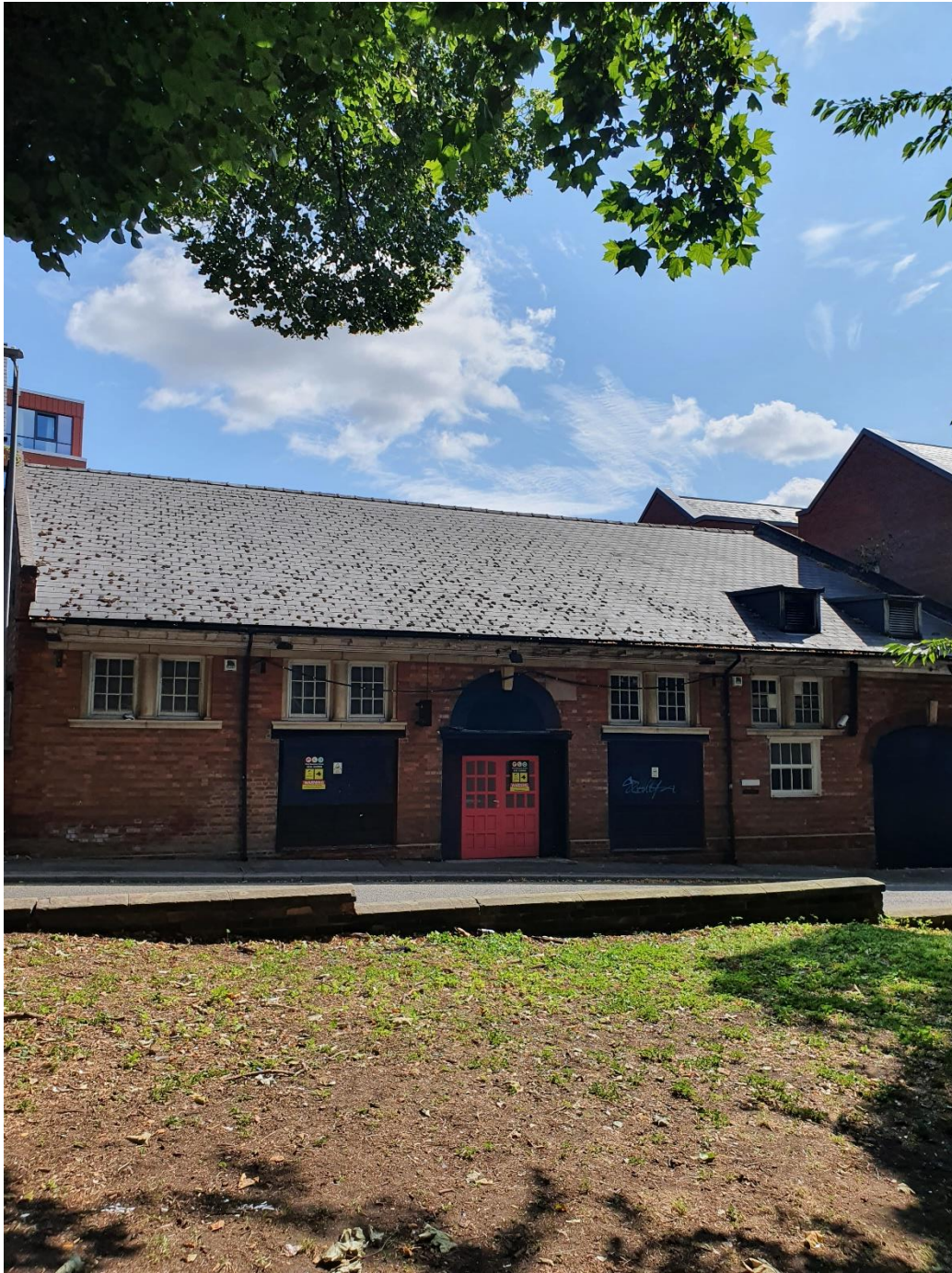
Todson House as existing
